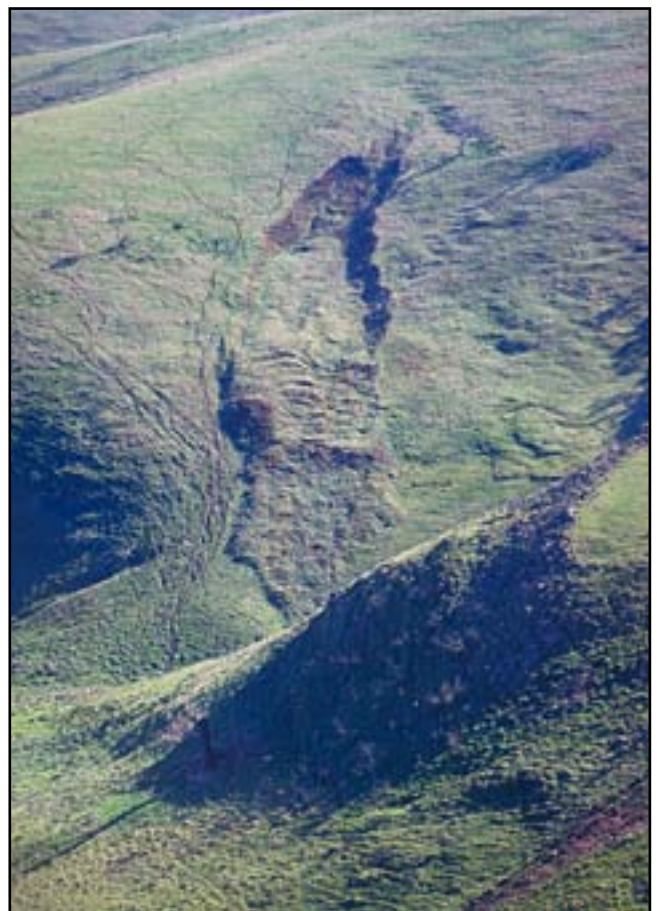
Little Para Dam. Talus slide at (20 degrees slope). Photo 012731
